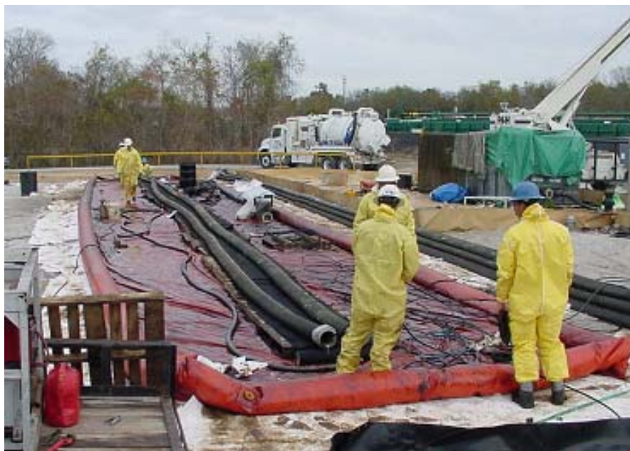
Figure 60 Final Hose Decon in Progress by the ASCO Crew.
