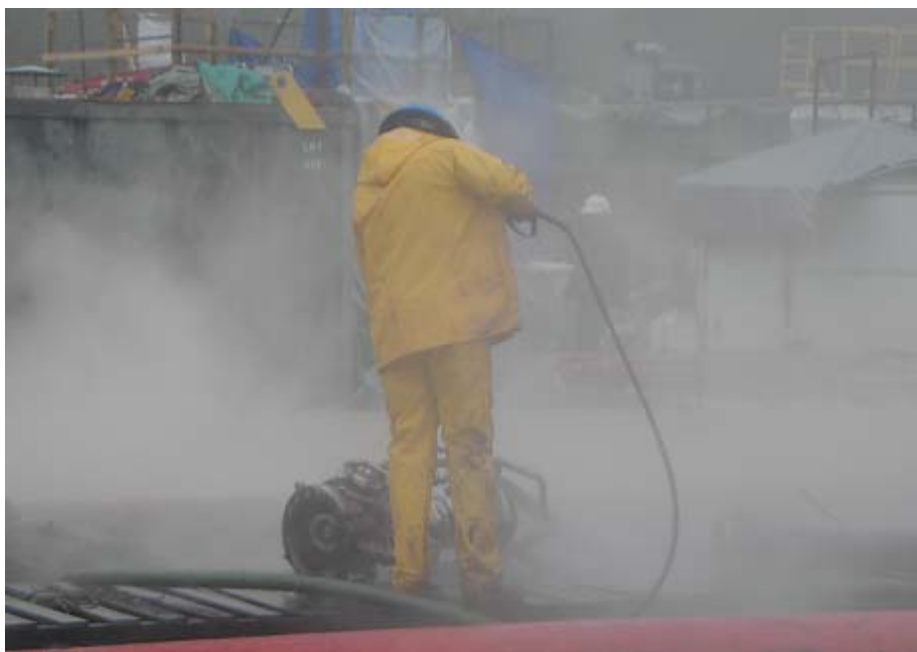
Figure 61 Equipment Decontamination in Progress, here of a DOP-250 pump.
