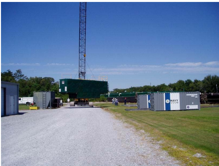
Figure 23 A Cenac Towing, Inc. Crane Lifts USCG 500 bbl Backup Tank into Position
