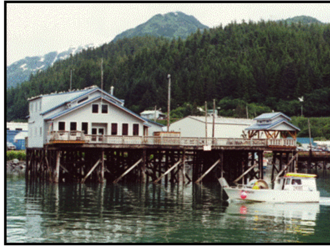
The Prince William Sound Science Center building located at the entrance of the harbor in Cordova, Alaska.
